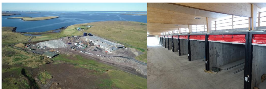
Figure 1. GAJA biogas and composting station
