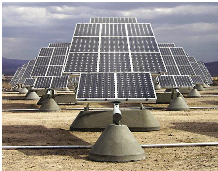
Figure 2. Photovoltaic system with portable crystalline panels with dual-axis tracker Source: from Frontier Associates, LLC (2008, p.3-18)
