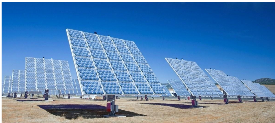
Figure 3. Photovoltaic system with concentrating portable panels with dual-axis tracker Source: from Schwartz (2008)
