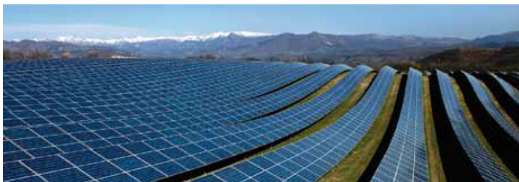
Figure 1. Photovoltaic system with rigid crystalline panels
